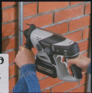
For drilling saddle joints for electrical conduit
