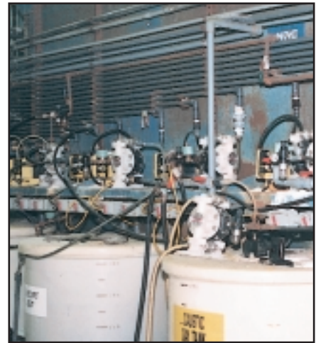
ARO 1/2" pumps being used in a water pre-treatment operation
