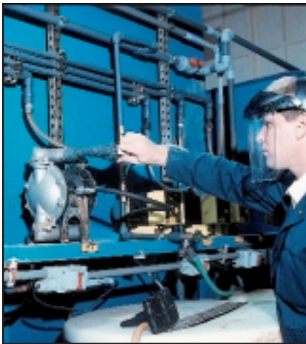
A 666101-244 (1" Stainless Steel) is used to supply water treatment chemicals
